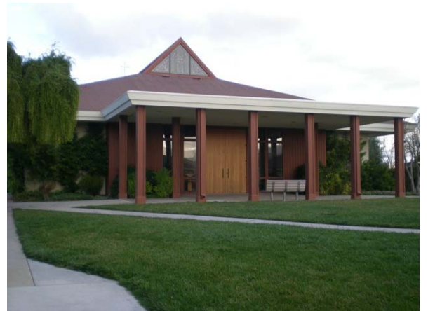
Sanctuary from the Church Quadrangle
